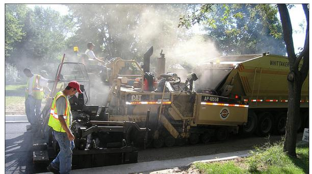
The picture above shows the hazardous release of PAHs (smoke) into the environment during the installation of Hot Mix Asphalt.
